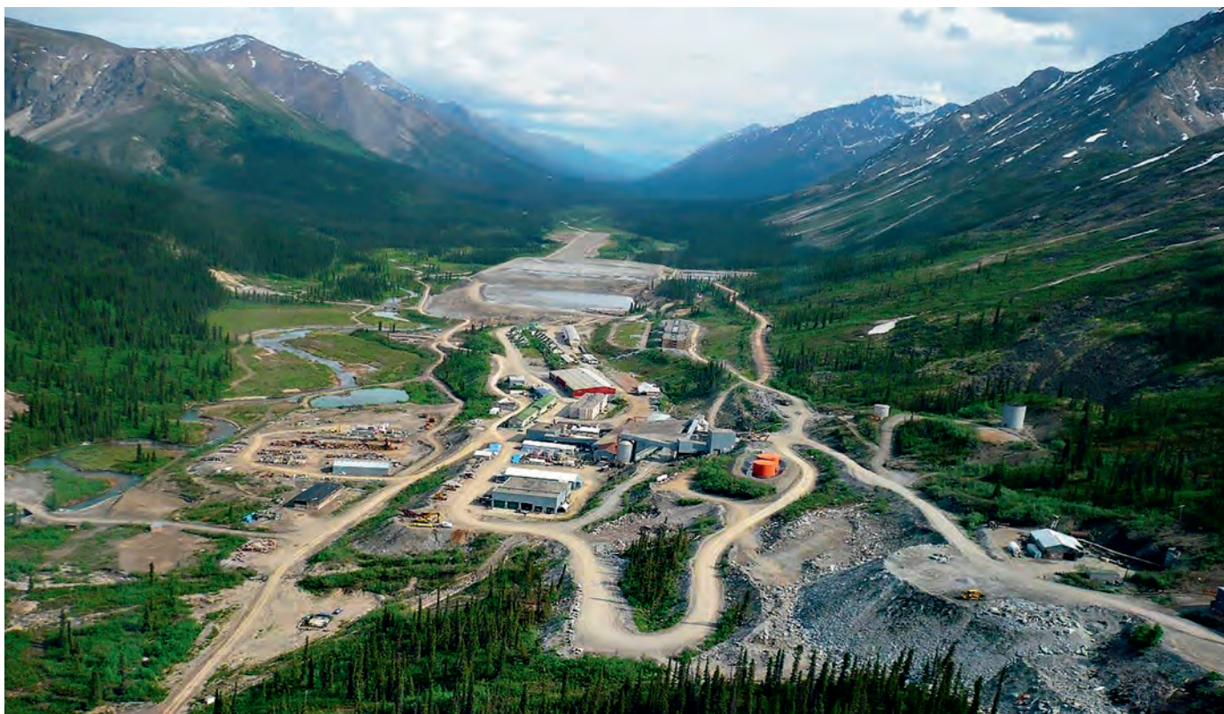
Aerial photo of the Cantung mine. Ore dressing plant in the foreground, tailings pond and air strip in the background
