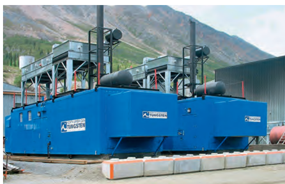
Power generators with heat recovery systems
